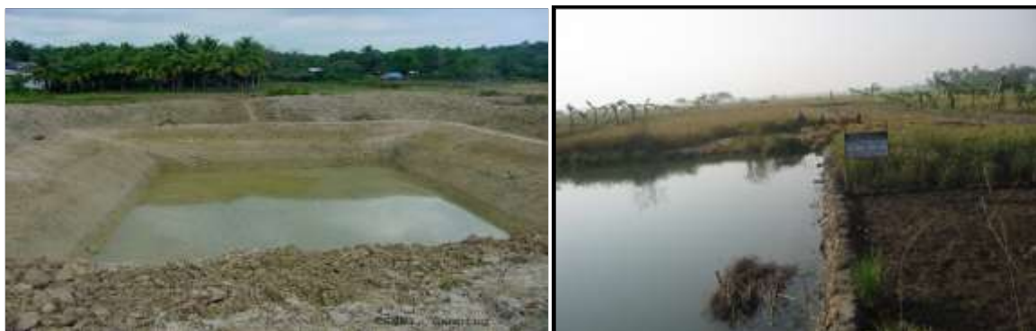
Fig. 1. farm pond excavation and land raising in the Farmers field
